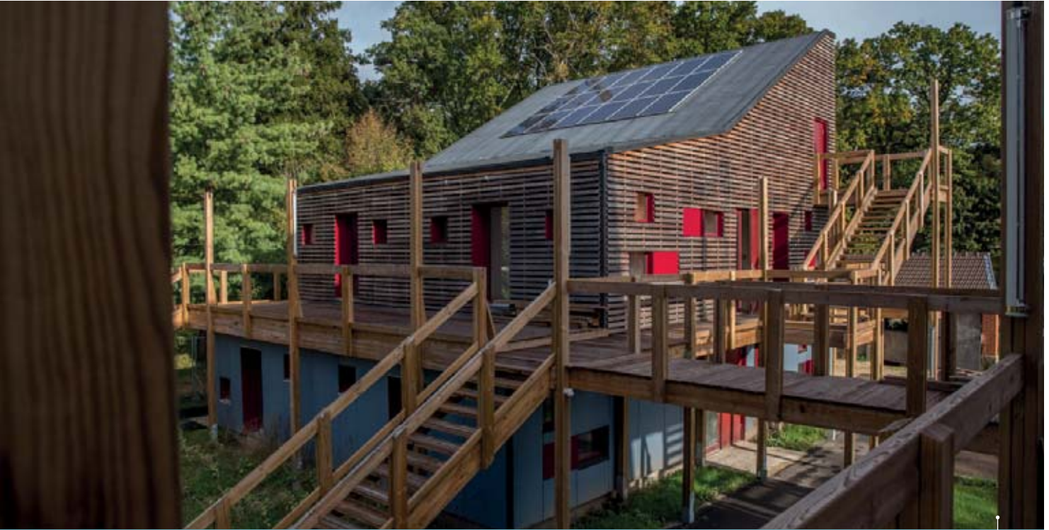
Timber-framed house with solar power, Bouray-sur-Juine, 91 - ©AREC
